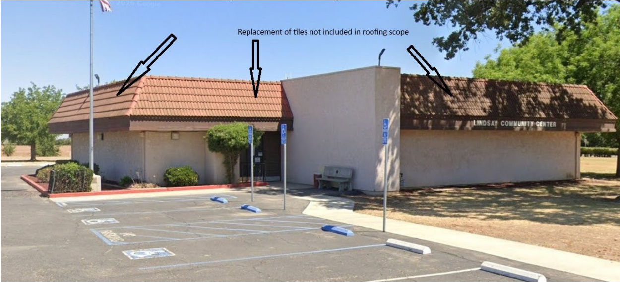
Figure C.7.2 Existing Roof Tiles
